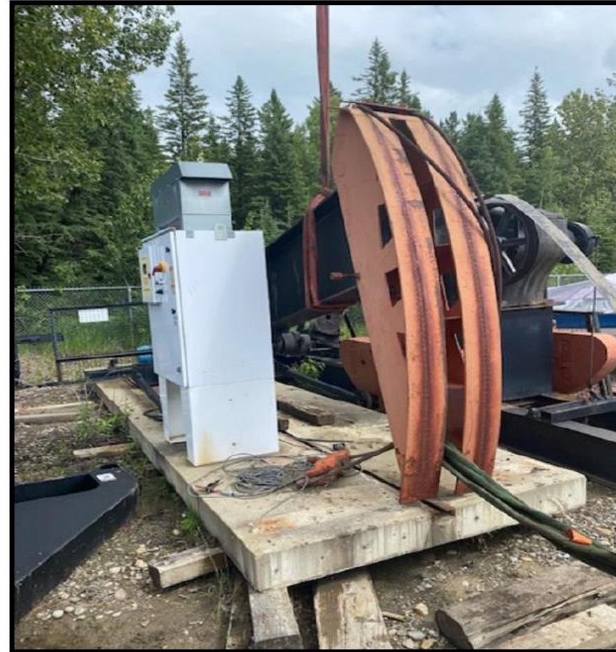
Image of the fallen equipment.
