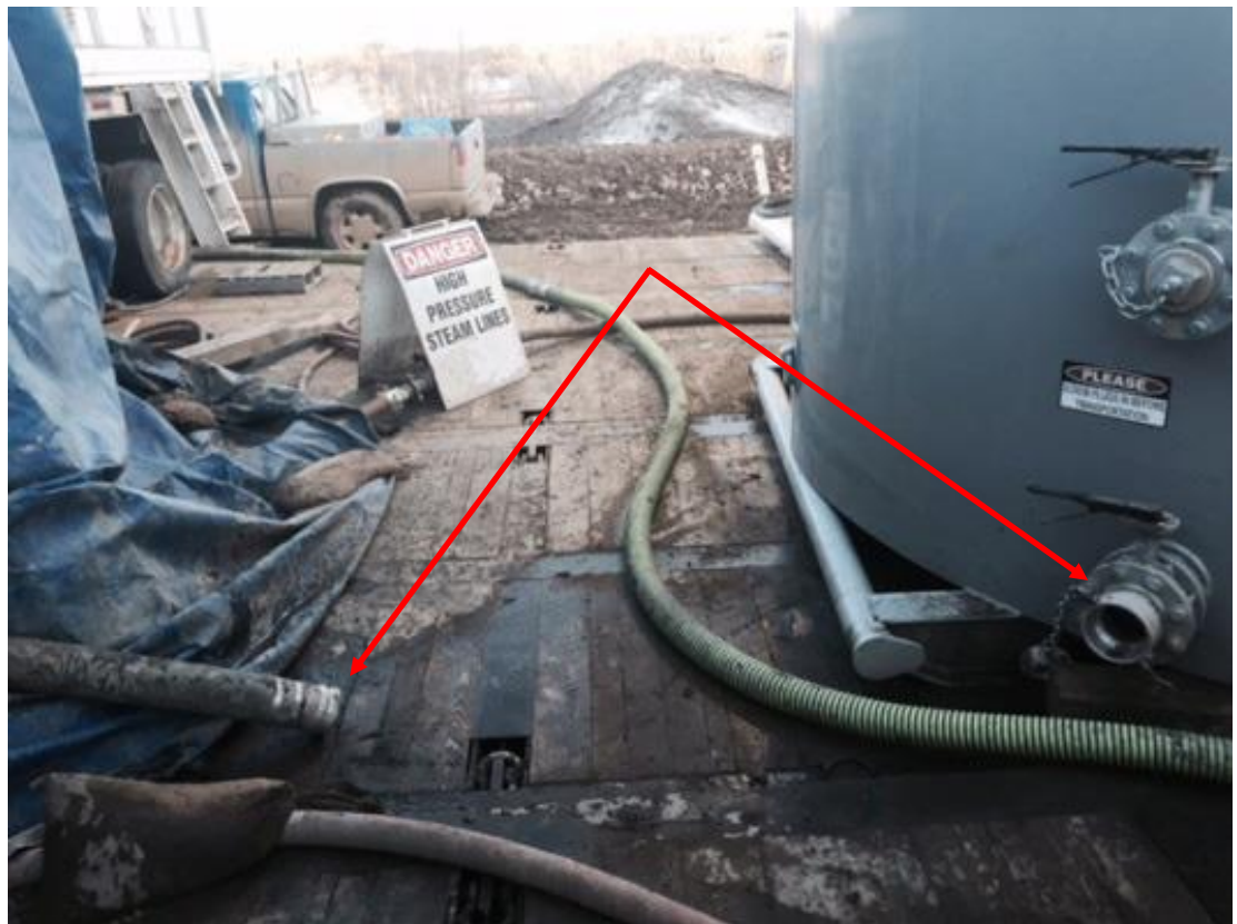
Arrows show location where hose landed and location on tank where hose was attached.
