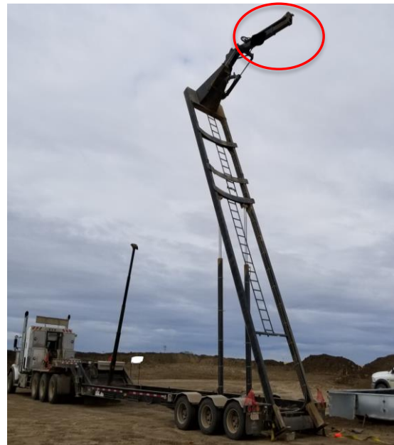
Failed bracket at the top of the tank cradle arm
