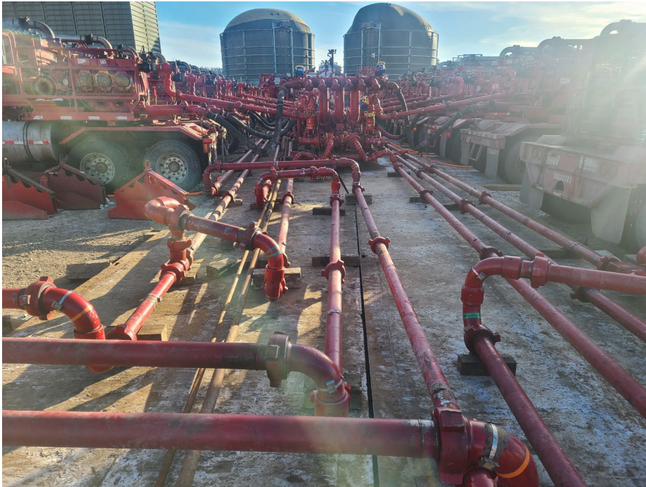
Figure 3. Hydraulic Fracturing Pipework System Before Restraint Application
