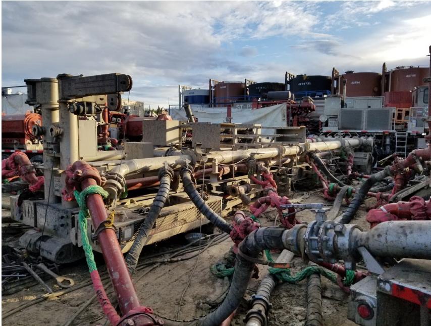
Figure 7. Discharge Iron from Fracture Pumpers to Manifold Trailer with Restraints
