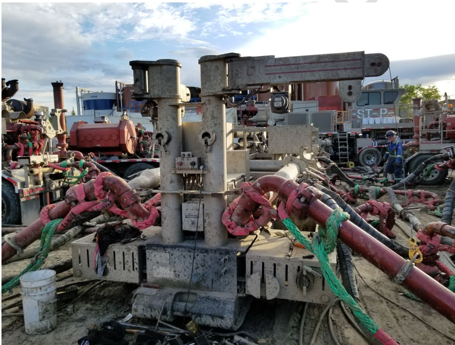
Figure 8. Discharge Iron from Fracture Pumpers to Manifold Trailer with Restraints
