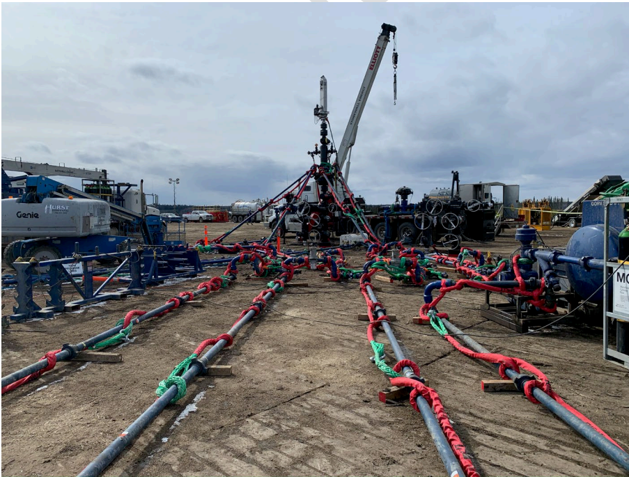
Figure 39. Restraint System
