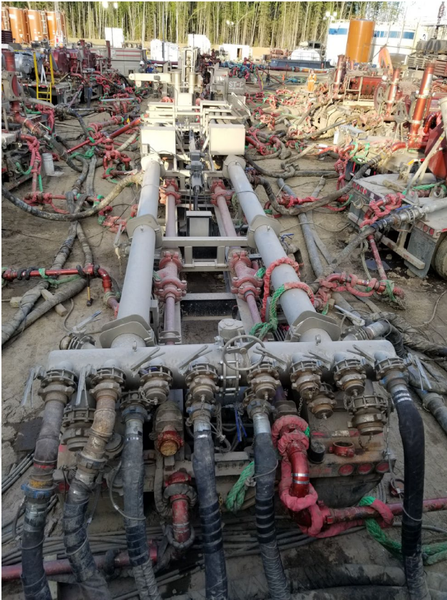
Figure 10. Discharge Iron from Fracture Pumpers to Manifold Trailer with Restraints
