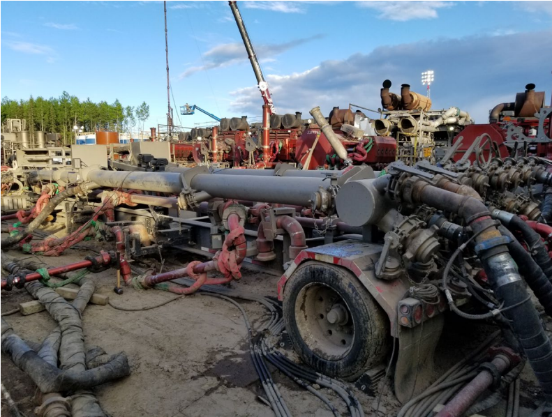
Figure 9. Discharge Iron from Fracture Pumpers to Manifold Trailer with Restraints
