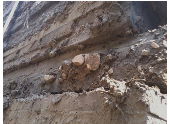
CLOSE-UP VIEW OF MUD AND ROCKS ATTACHED TO MATTING
