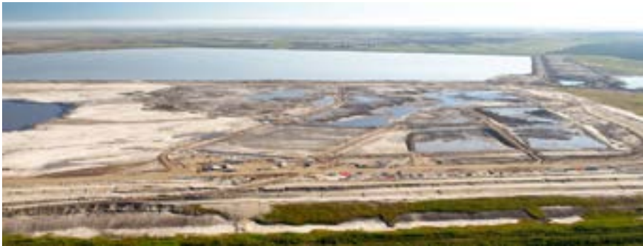
Image 1: Aerial photo of an oil sands tailings storage facility.
