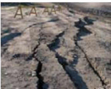
Cracking or sliding along the crest
