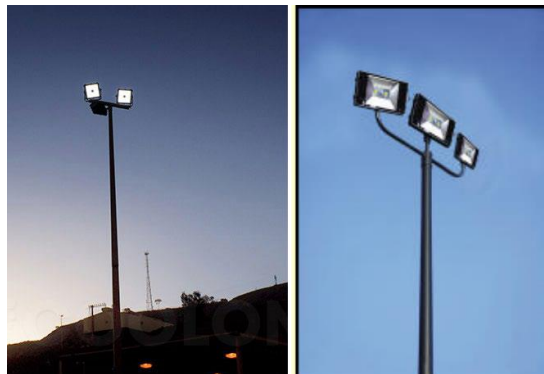
Figure E-7, E-8, E-9: LED floodlights (140 watt floodlight version replaces a traditional 450 watt bulb)
