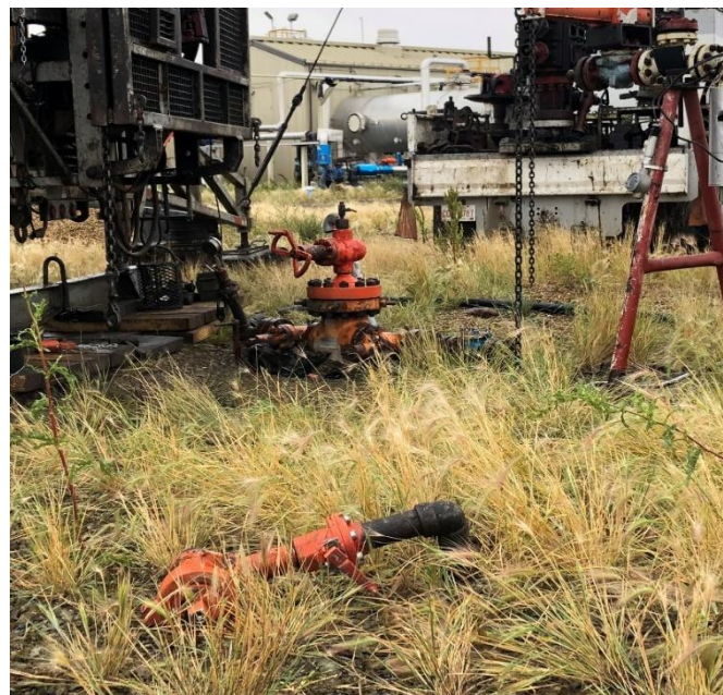
Image of Flow 'T' and wellhead (post incident)
