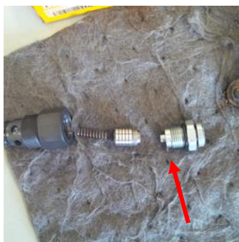
The orifice was rebuilt in the improper order, as it was installed in the main valve.
