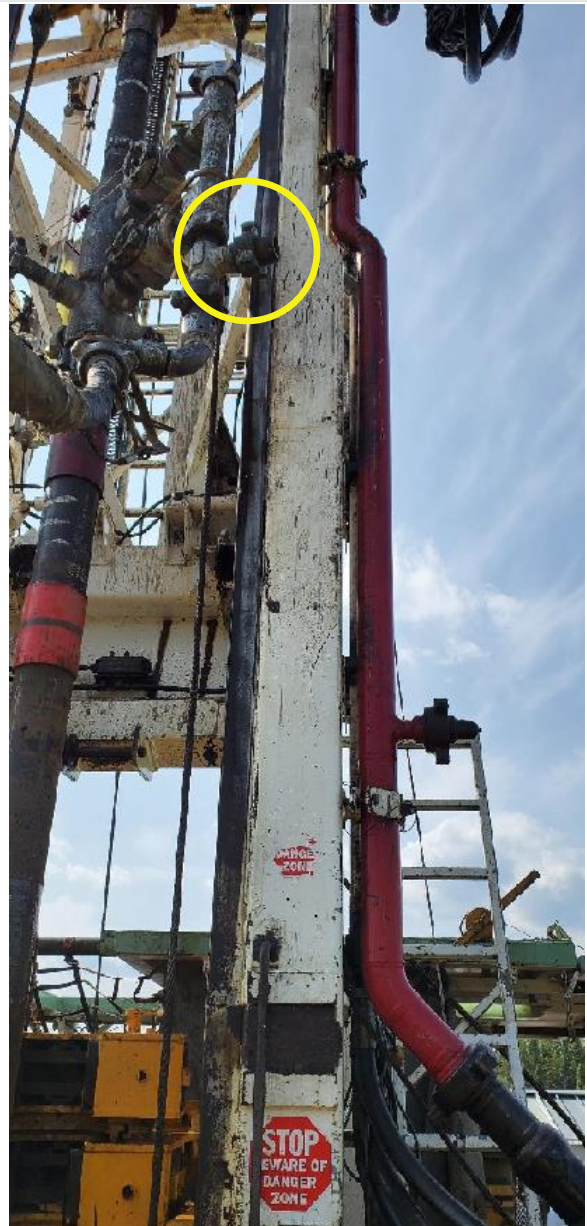
Location of the point of failure at the time of the incident
