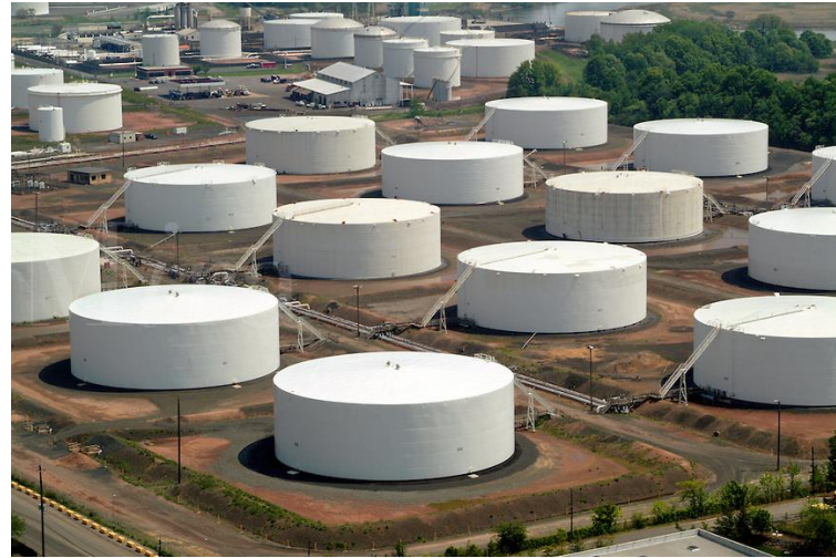
Example of a typical tank farm
